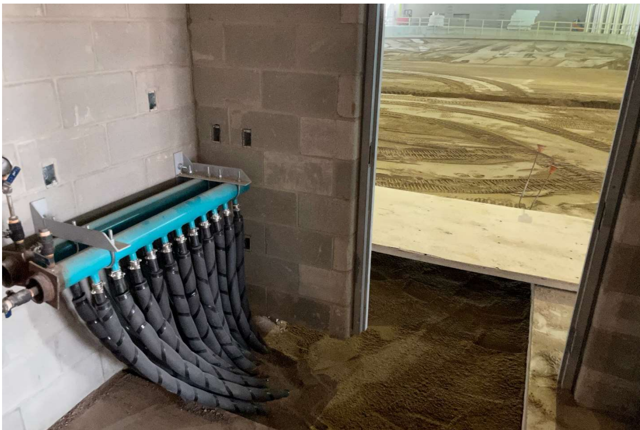
Arena 1 – Under Slab Heat Piping and Sand Installation Complete
