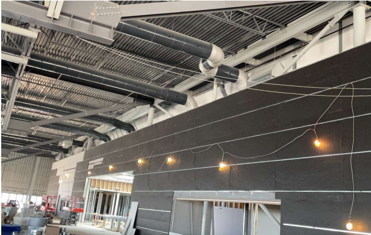
Gymnasium – Installation of HVAC Ductwork, Drywall, Acoustic Panels
