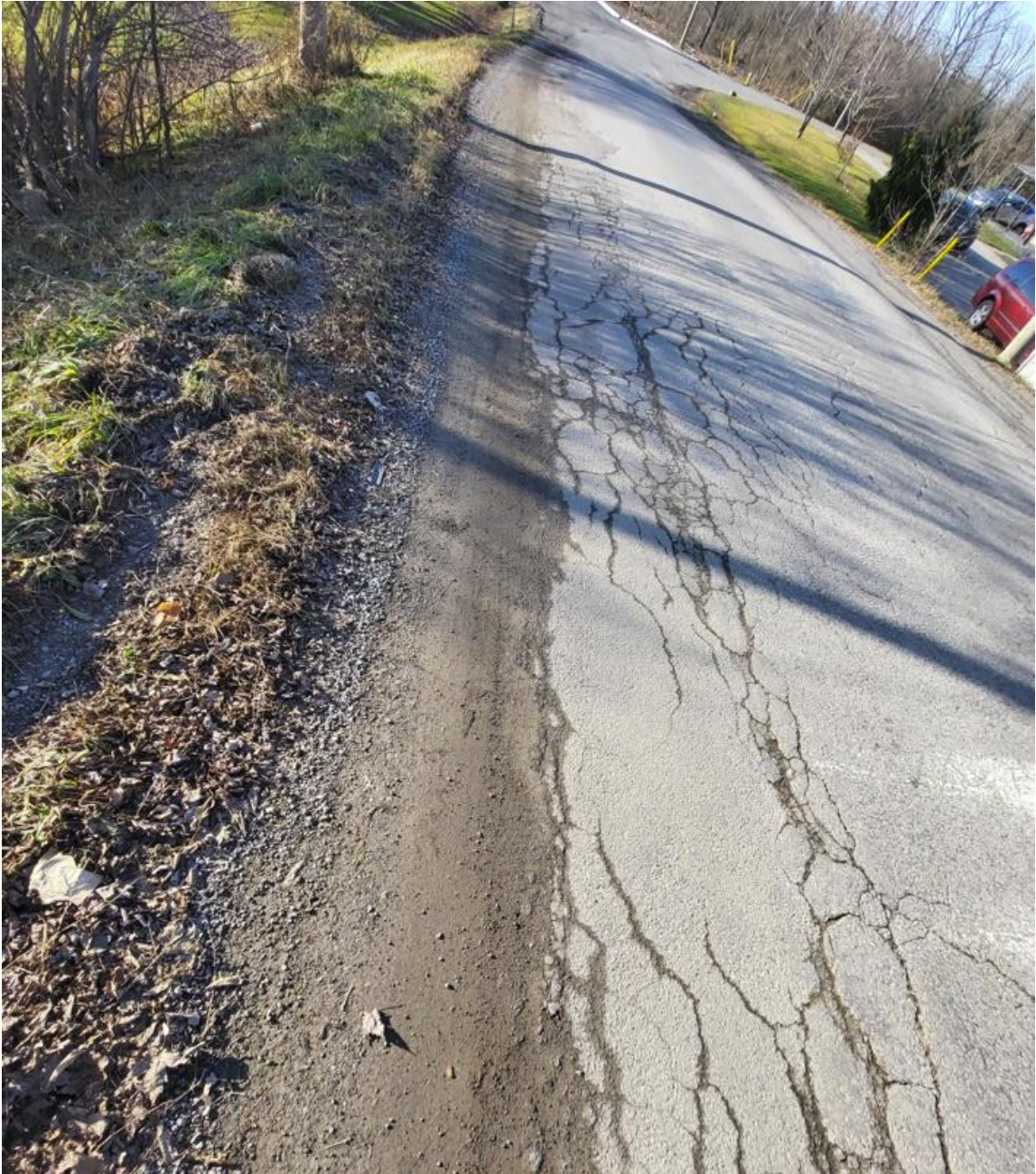
Figure C-5: Barron Road (West) Crossing – Shoulder Condition
