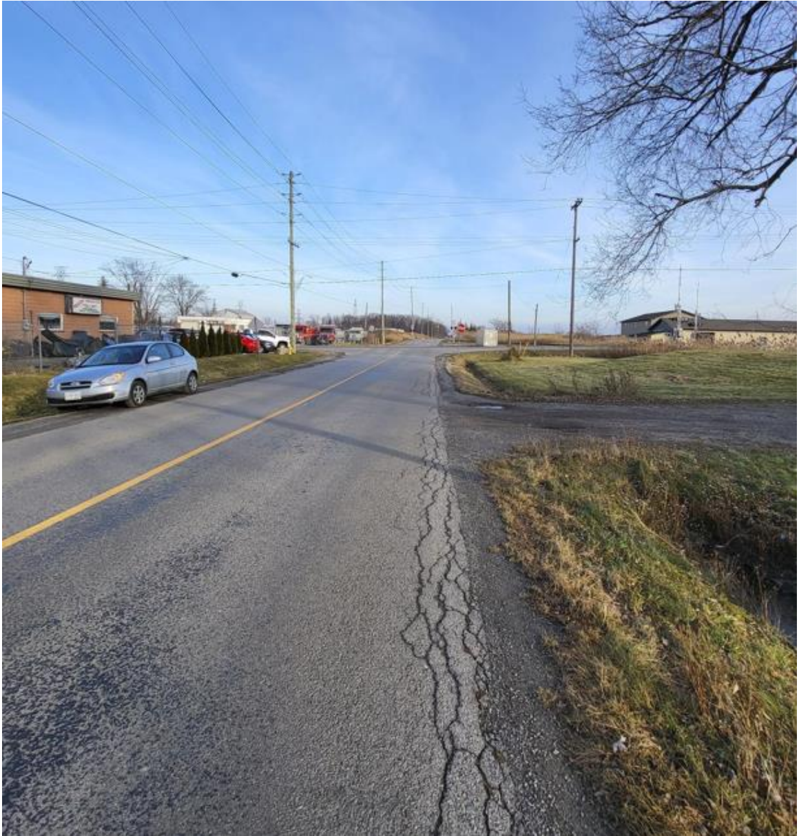
Figure D-6: Barron Road (East) Crossing Sightline Visibility – Eastbound Approach (105m)
