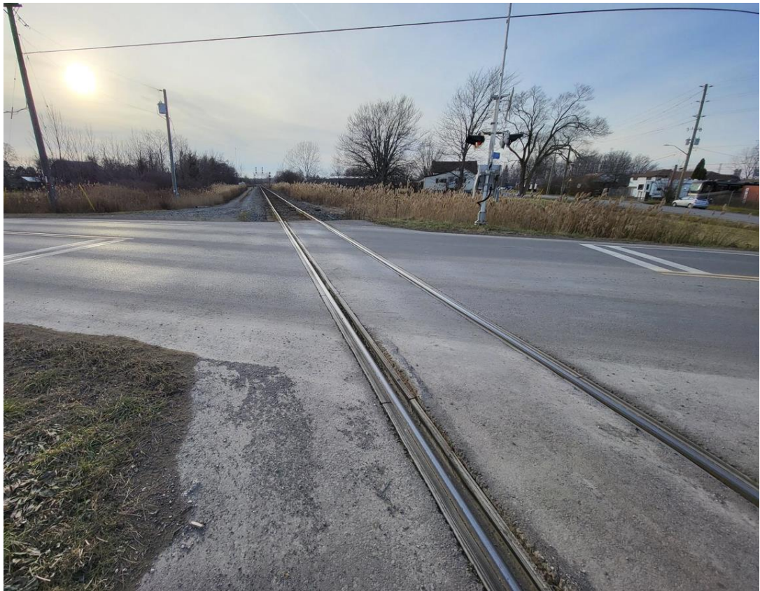
Figure E-16: Allanport Road Crossing – Grade Crossing Surface (Facing Westbound)
