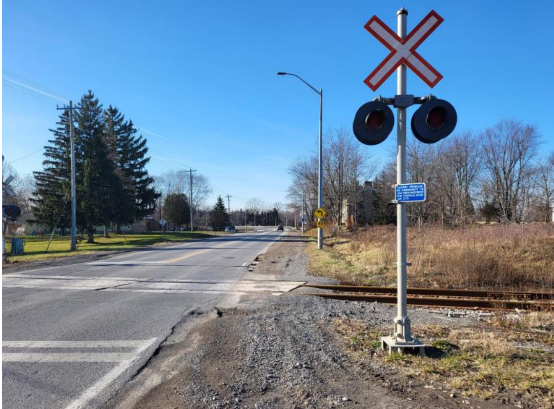
Figure A-18: Lundy's Lane Crossing – Warning System
