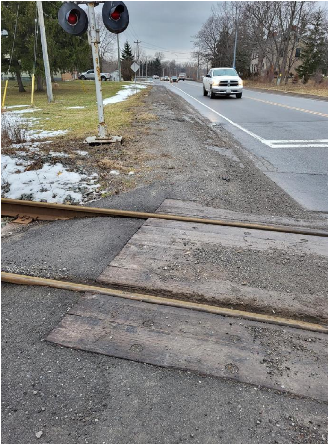
Figure A-3: Grade Crossing Surface (South side)
