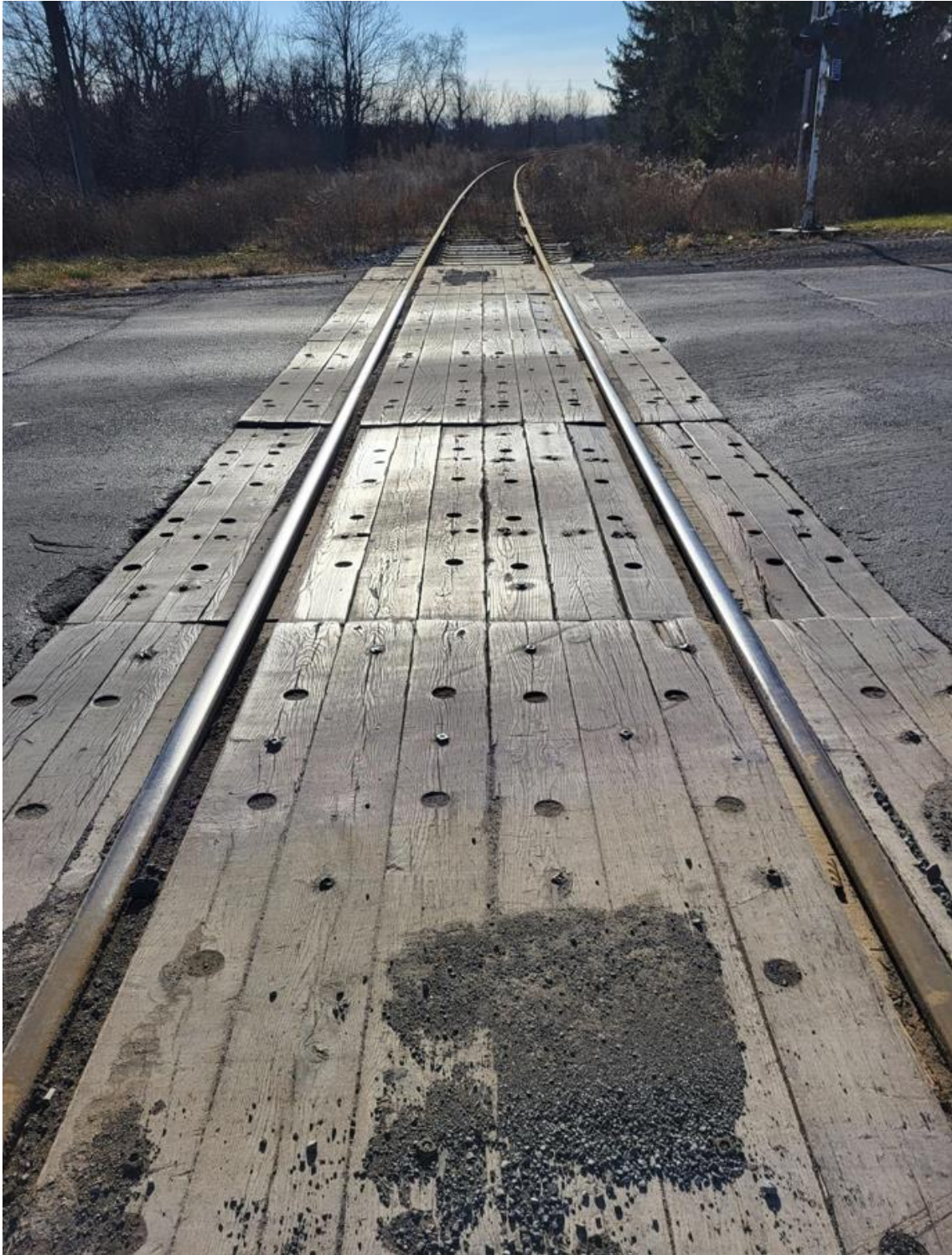
Figure A-1: Lundy's Lane Crossing – Crossing Material
