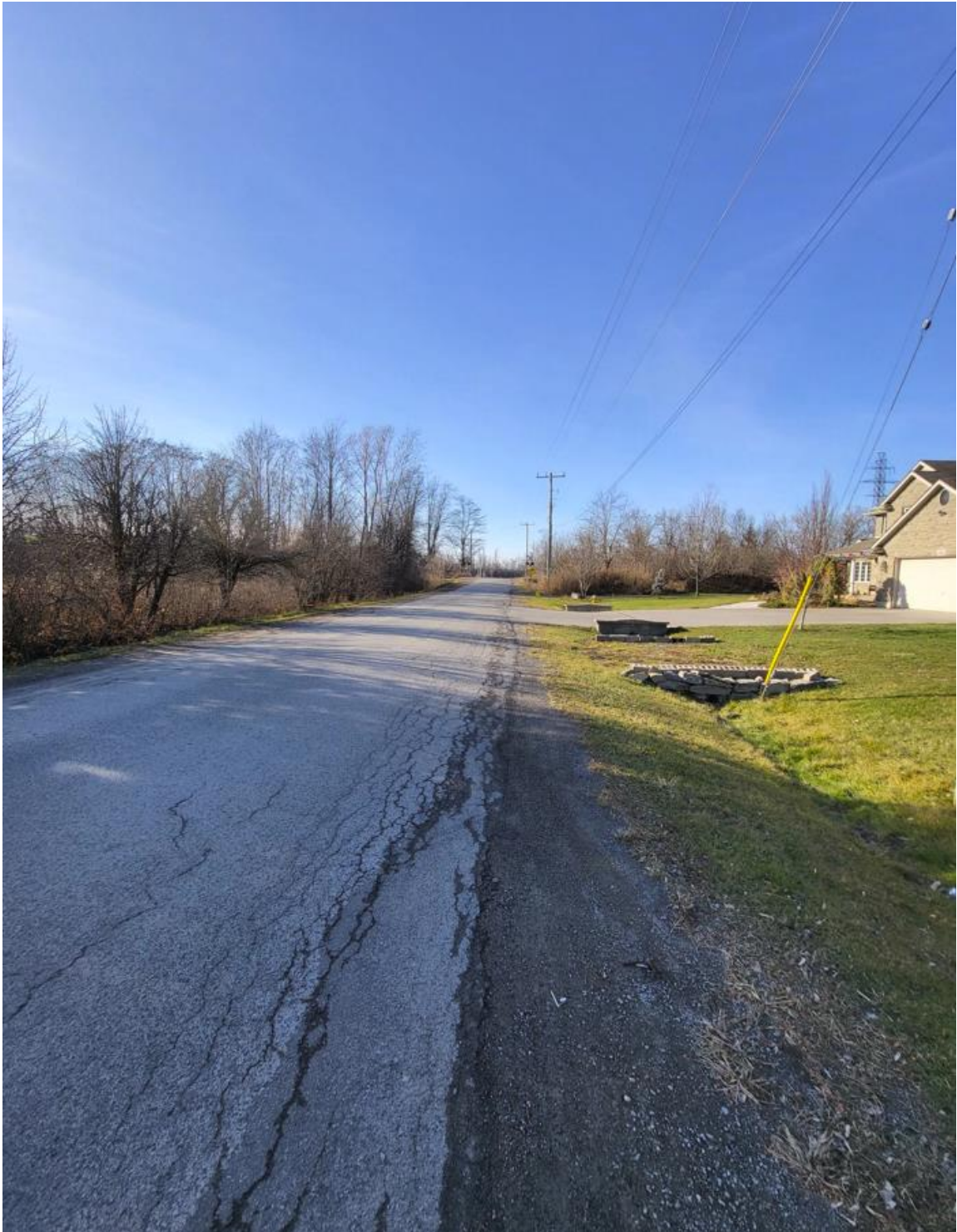
Figure C-6: Barron Road (West) Crossing Sightline Visibility – Westbound Approach (85m)
