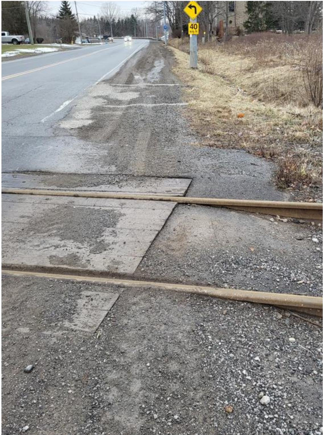
Figure A-2: Grade Crossing Surface (North side)
