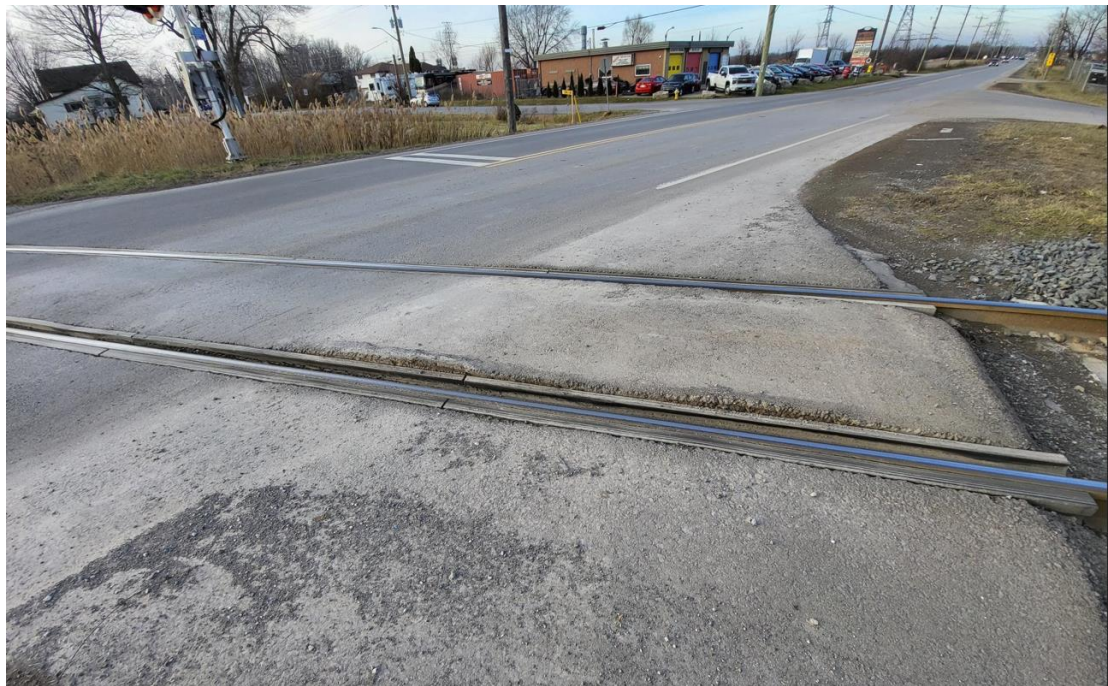
Figure E-3: Allanport Road Crossing – Grade Crossing Surface (Facing Northbound)
