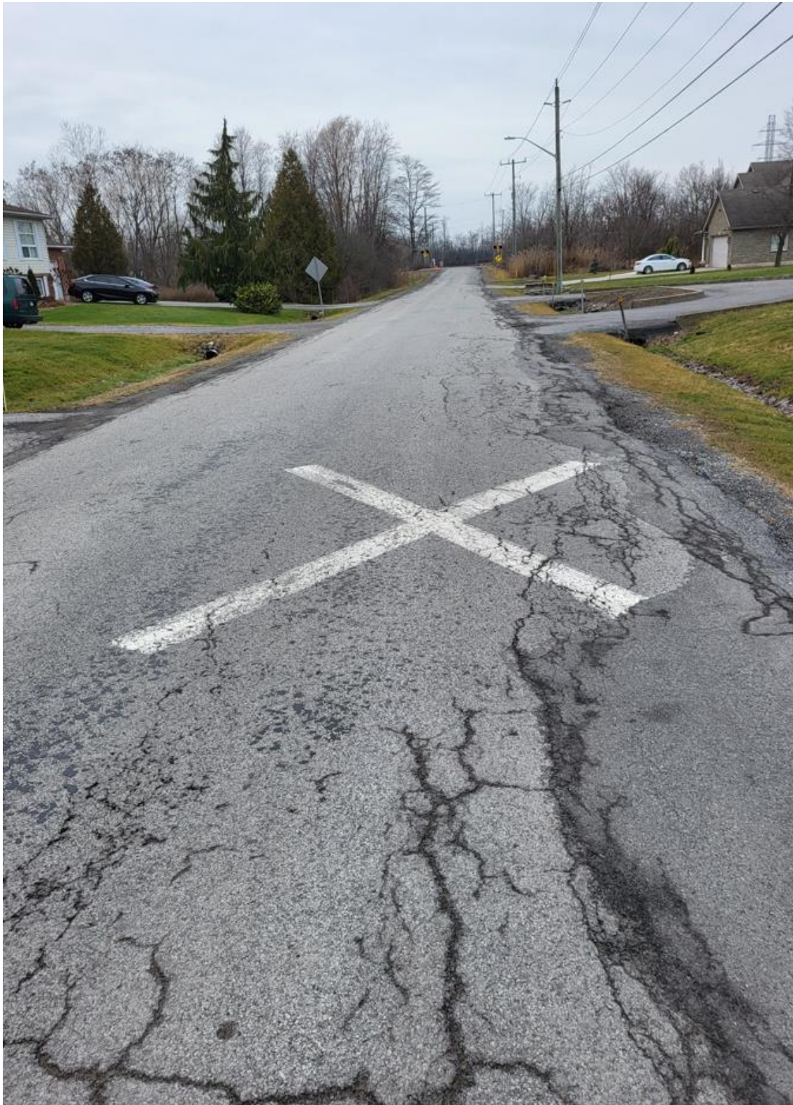
Figure C-13: Barron Road (West) Crossing – View from painted “X” (Westbound Approach)
