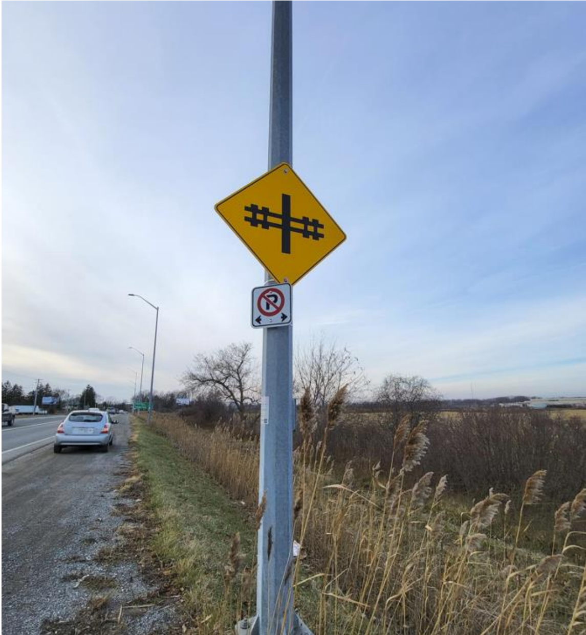
Figure A-12: Lundy's Lane Crossing Warning Signage – Westbound Approach
