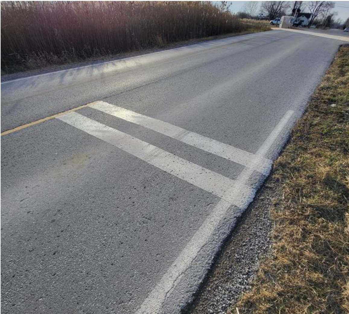
Figure D-10: Barron Road (East) Stop Bar – Westbound Approach
