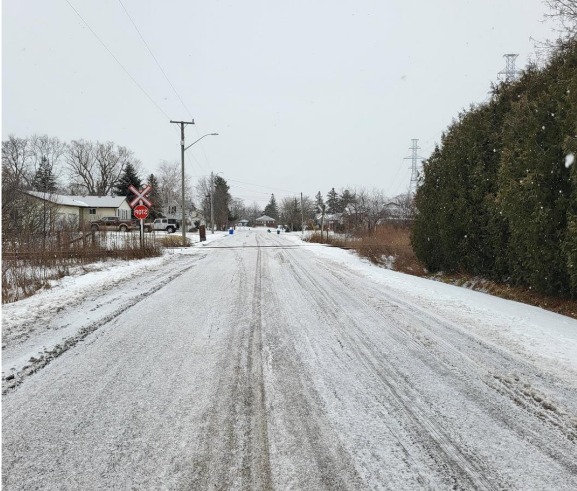
Figure B-3: Henderson Street Crossing Sightline Visibility – Westbound Approach (20m)
