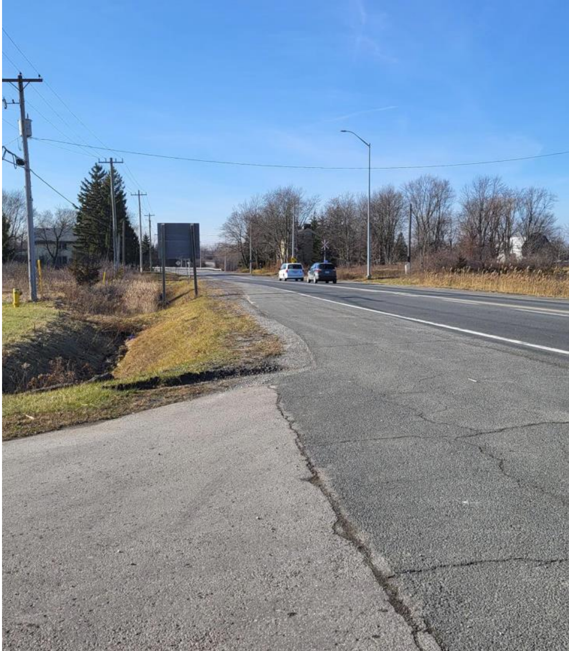
Figure A-17: Lundy's Lane Crossing – View from 13227 Lundy's Lane
