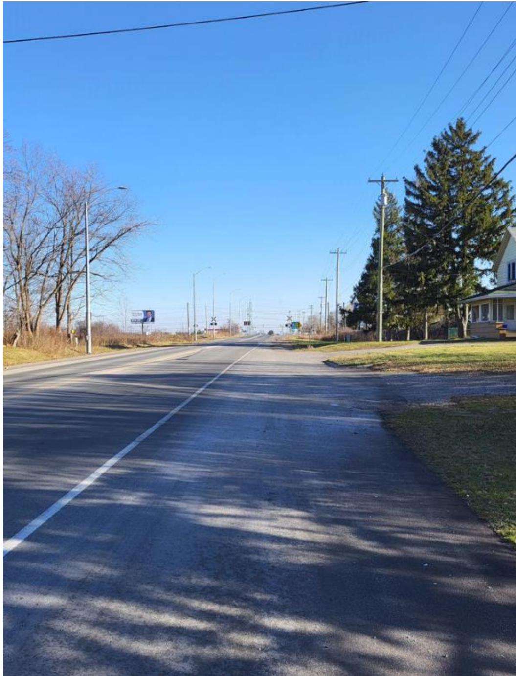
Figure A-5: Lundy's Lane Crossing Sightline Visibility – Eastbound Approach (105m)
