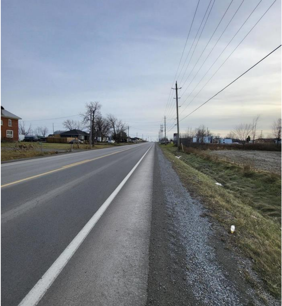
Figure E-5: Allanport Road Crossing Sightline Visibility – Southbound Approach (180m)
