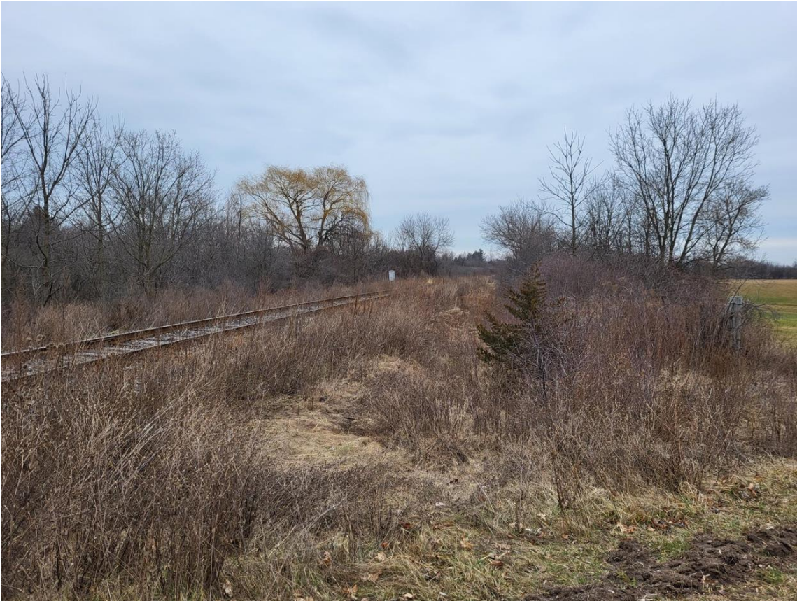
Figure B-8: Henderson Street Crossing (Dstopped) – Eastbound Approach (facing northbound)
