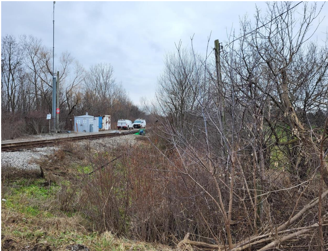
Figure C-8: Barron Road (West) Crossing (Dstopped) – Eastbound Approach (facing southbound)
