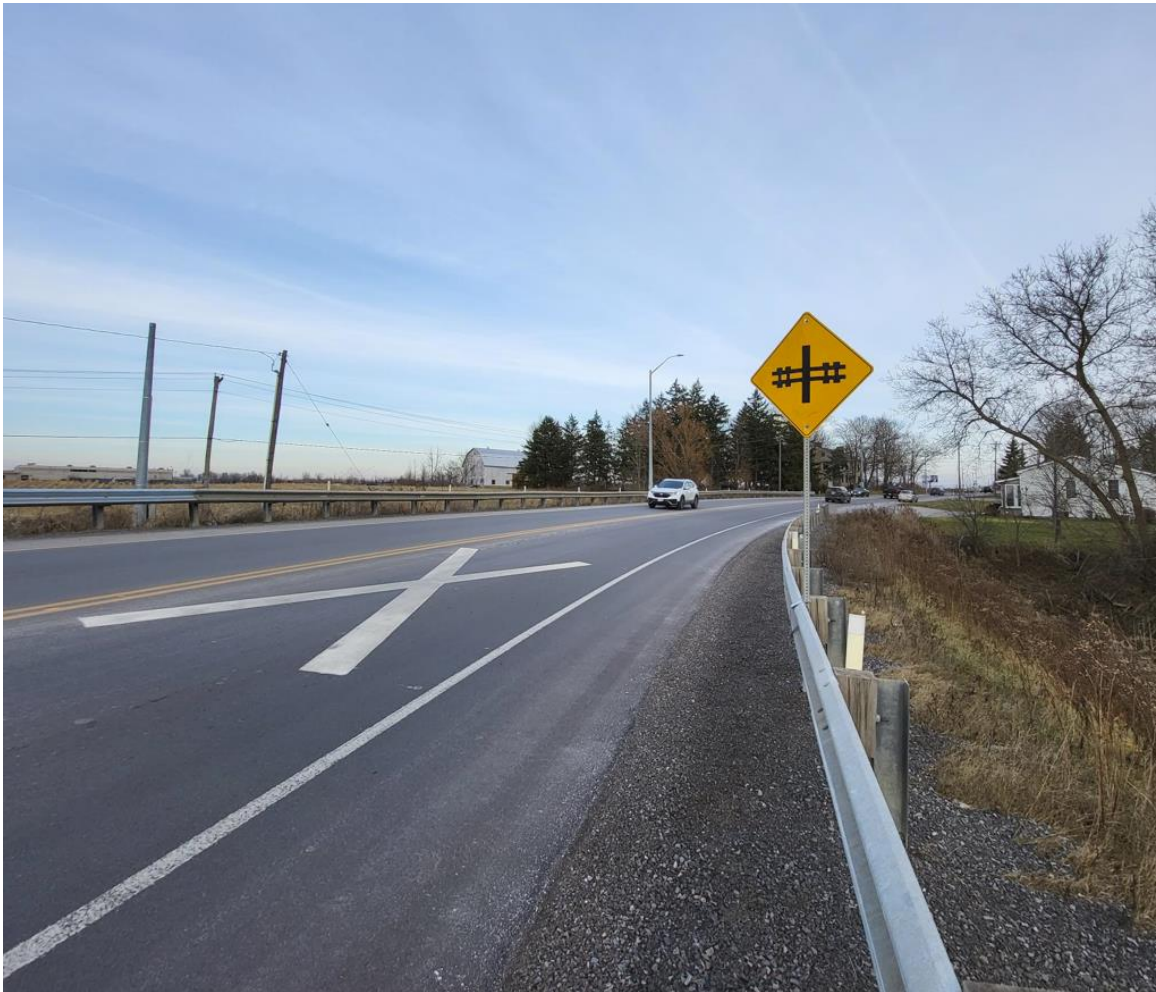
Figure A-13: Lundy's Lane Crossing Painted "X" and Warning Signage – Eastbound Approach
