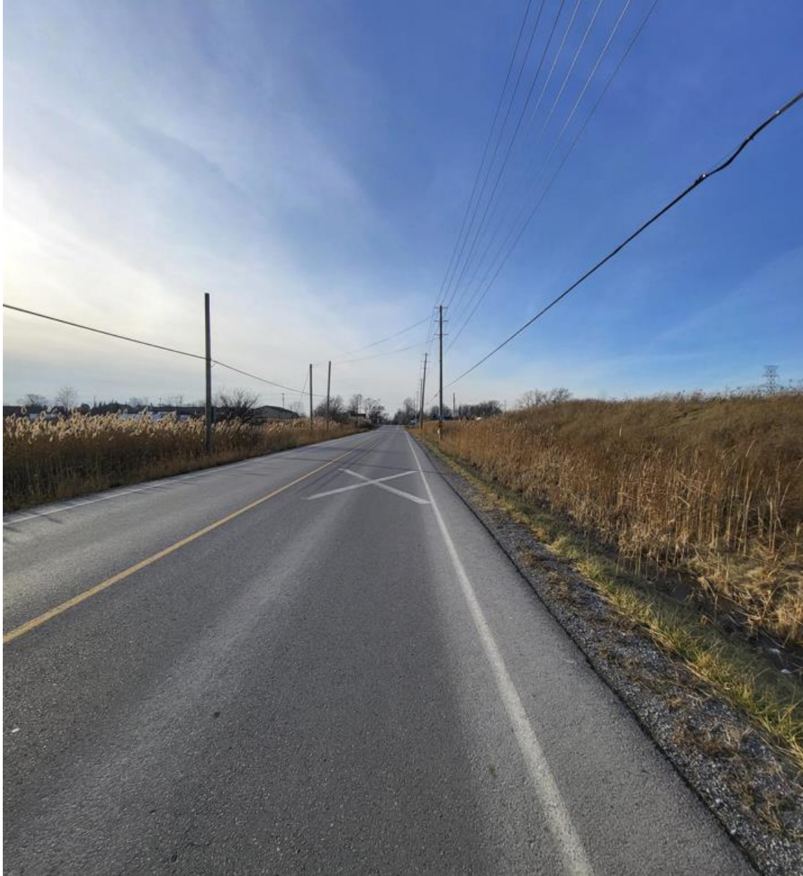
Figure D-5: Barron Road (East) Crossing Sightline Visibility – Westbound Approach (105m)
