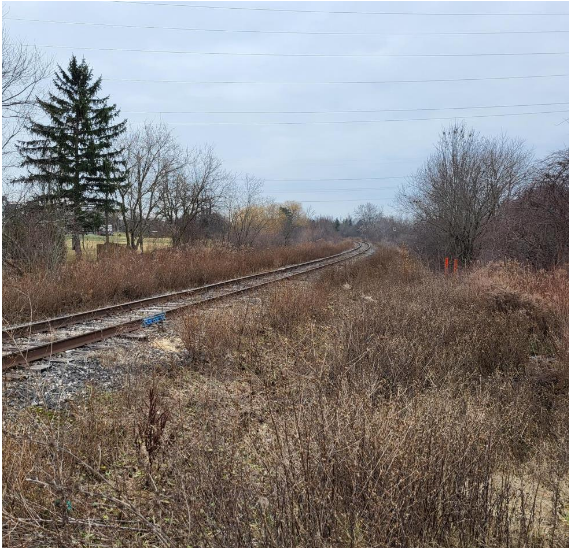
Figure B-5: Henderson Street Crossing (Dstopped) – Eastbound Approach (facing southbound)
