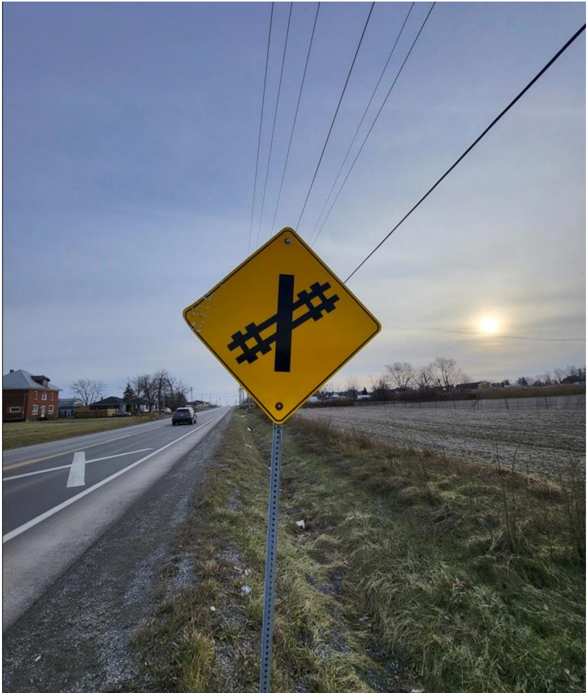
Figure E-8: Allanport Road Crossing Warning Sign Condition – Southbound Approach (Front of Sign)
