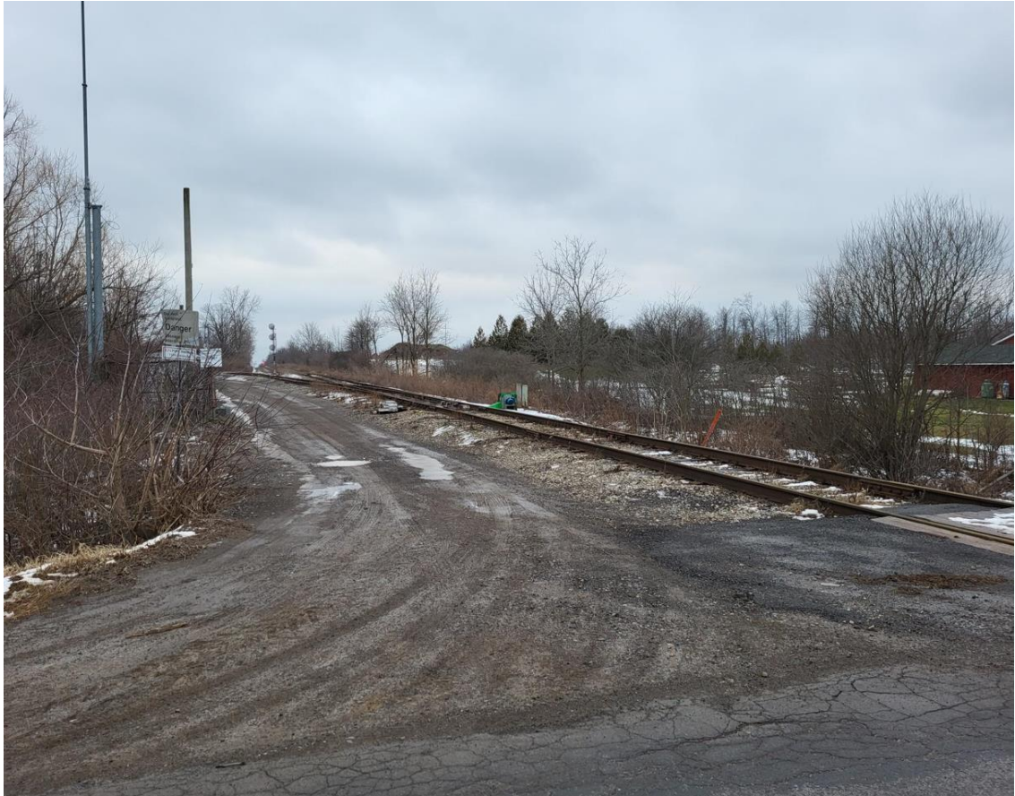
Figure C-11: Barron Road (West) Crossing (Dstopped) – Westbound Approach (facing southbound)
