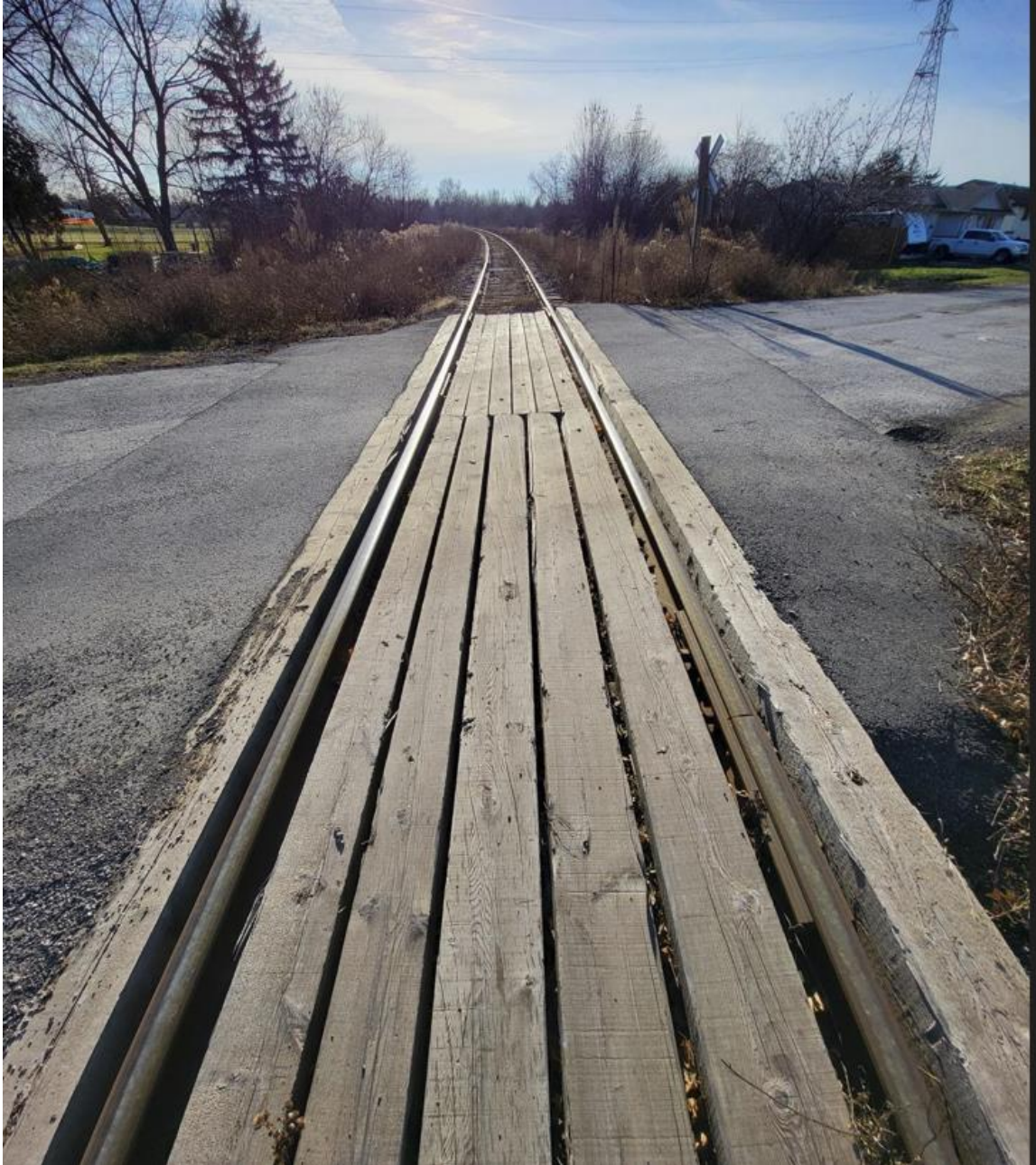
Figure B-1: Henderson Street Crossing – Crossing Material
