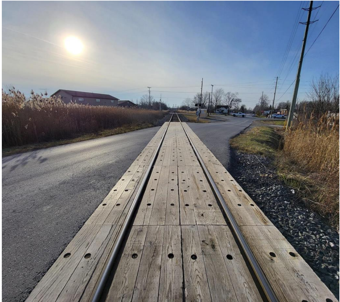
Figure D-3: Barron Road (East) – Crossing Material
