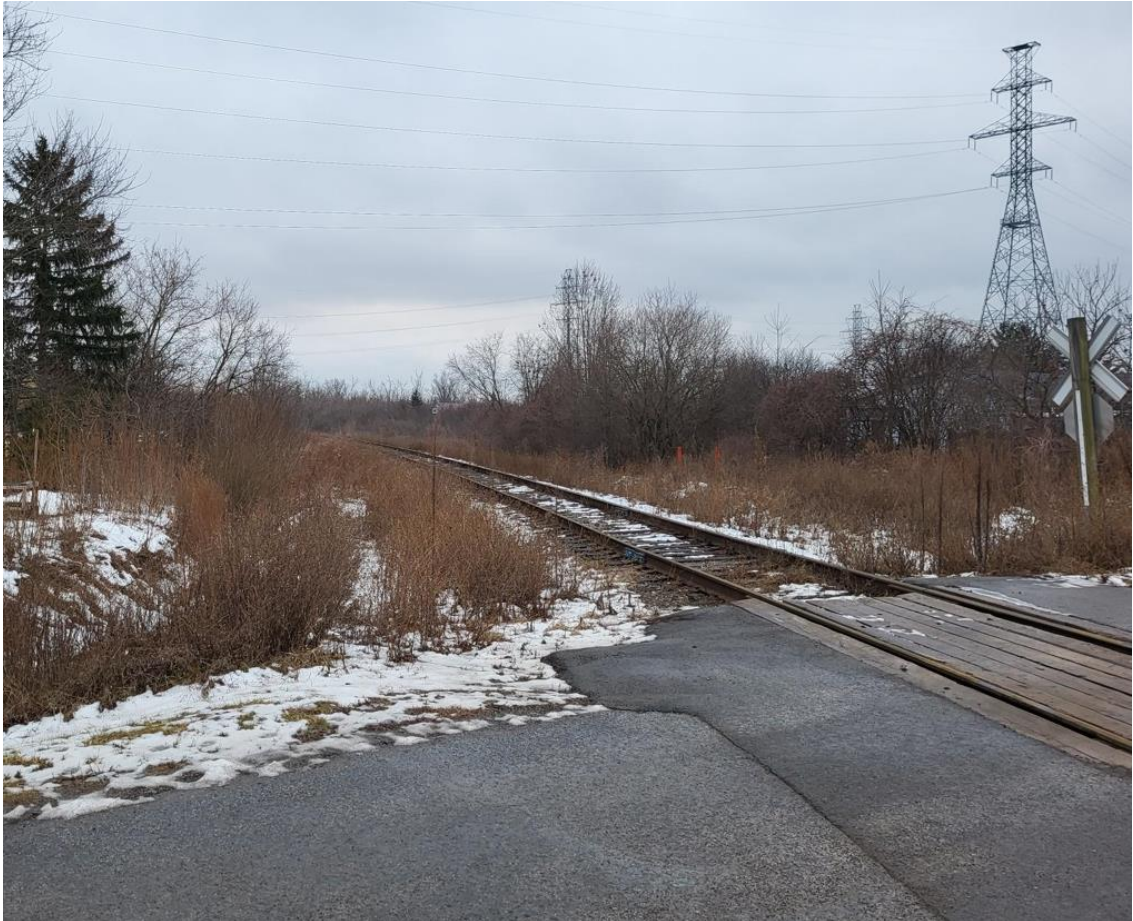
Figure B-7: Henderson Street Crossing (Dstopped) – Westbound Approach (facing southbound)
