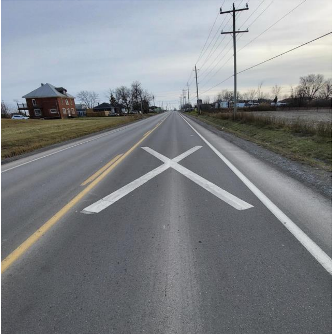
Figure E-15: Allanport Road Crossing Southbound Approach – Painted “X”
