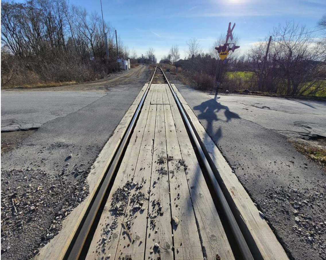
Figure C-4: Barron Road (West) Crossing – Crossing Material
