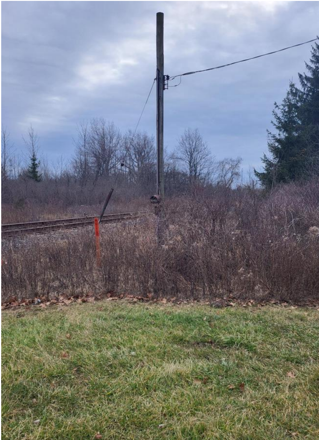
Figure A-9: Lundy's Lane Crossing Dstopped (eastbound approach facing southbound) – 50m
