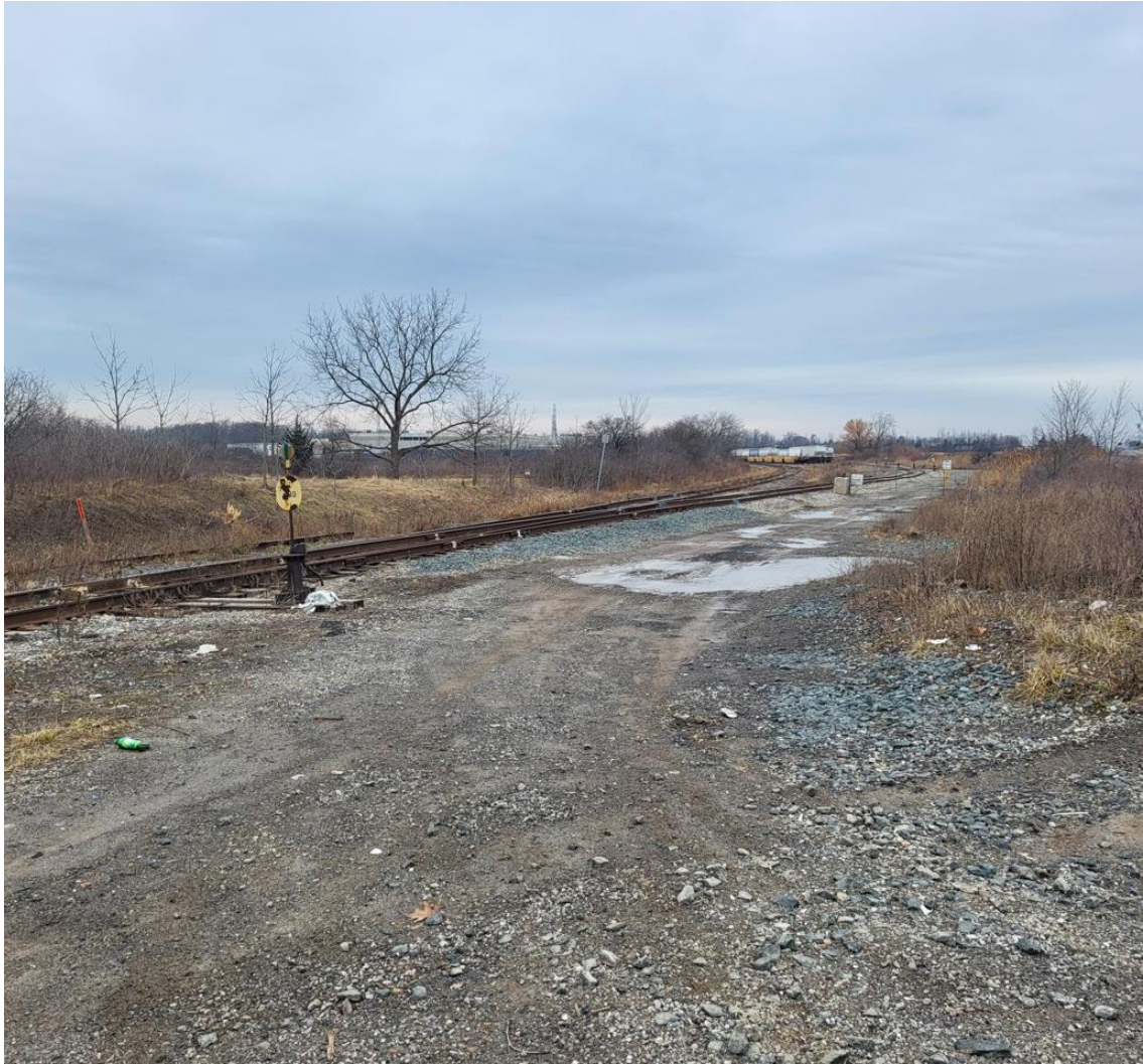
Figure A-7: Lundy's Lane Crossing Dstopped (westbound approach facing southbound) – 50m
