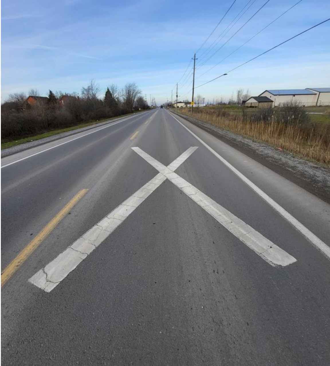
Figure E-14: Allanport Road Crossing Northbound Approach – Painted “X”
