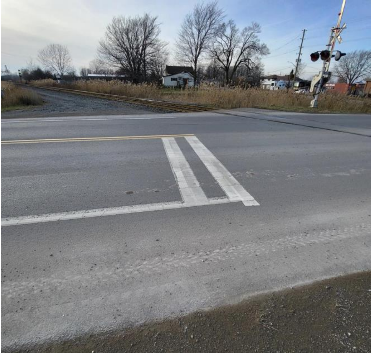
Figure E-12: Allanport Road Crossing Stop Bar – Northbound Approach
