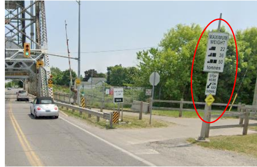
LUNDY LANE (RR20) LOOKING EAST AT WELLDAN CANAL TRAIL
