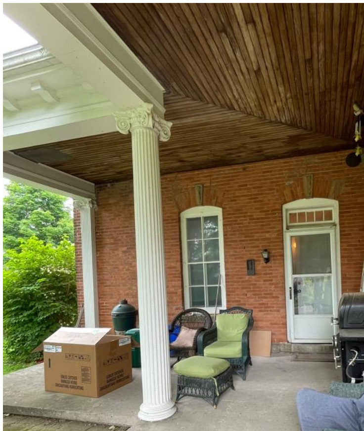
Northwest corner of house, beneath verandah
