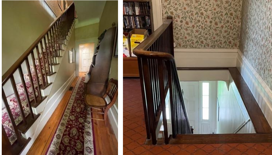
Central staircase (views from main floor and second-floor landing)
