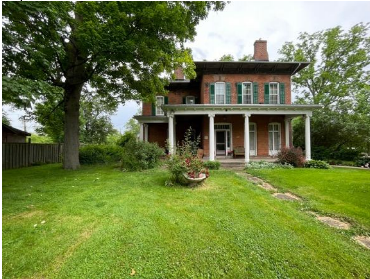
West-facing façade of 18 River Street
