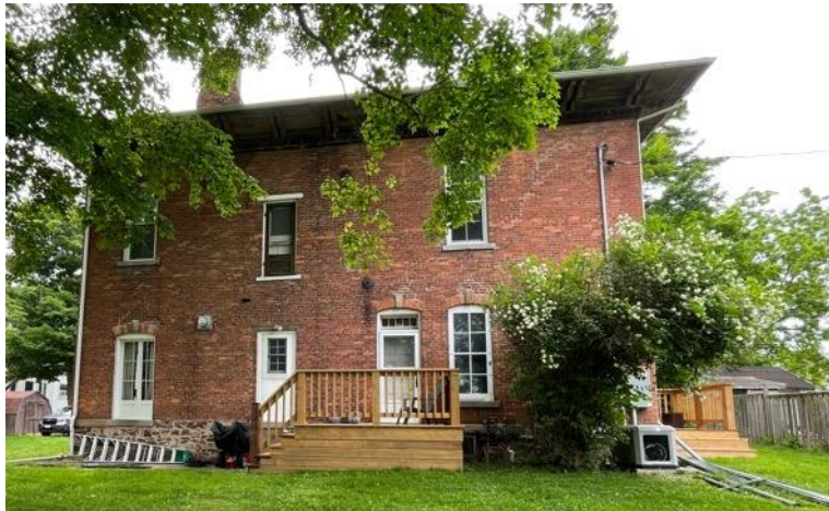
Rear (east facing) elevation
